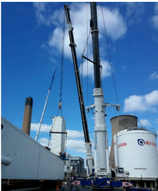
LIFT OF RECTIFICATION TOWER IN PREPARATION FOR LOADING READY FOR TRANSPORTATION TO COLESHILL
