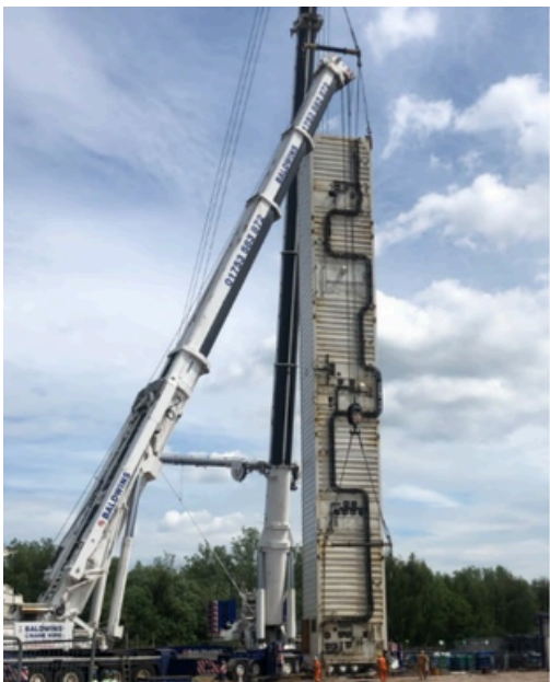
LIFT OF RECTIFICATION TOWER IN PREPARATION FOR LOADING READY FOR TRANSPORTATION TO COLESHILL
