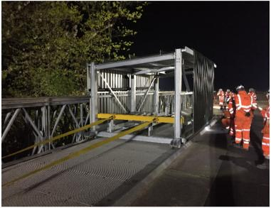
Three significant crossings were incorporated into the design of the conveyor layout. Firstly, a bridge designed and supplied by Mabey was launched over the railway line. Hargreaves conveyor sections had to fit directly onto the structure; this involved a bespoke winching system whereby the sections were pulled into place during a limited night-time rail possession.
