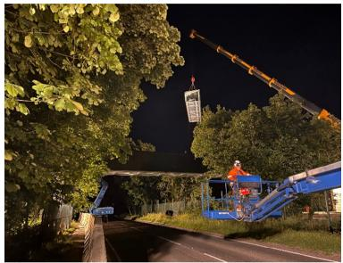
The two road crossings were also completed during nighttime road closures and involved a complex lift as the modular sections were craned into place onto pre-installed trestles supplied as part of the design.
