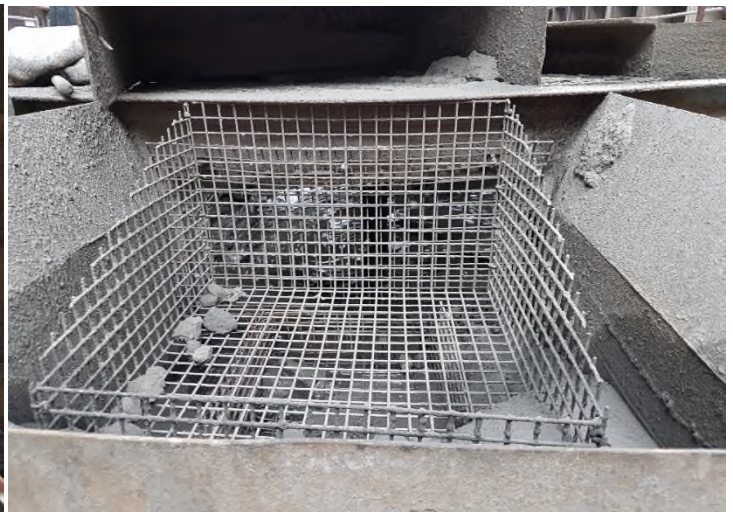
Figure.2 – mesh baskets fitted to receiving tanks
