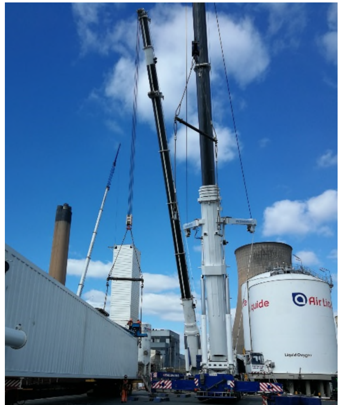
Lift of Rectification Tower in preparation for loading ready for transportation to Coleshill
