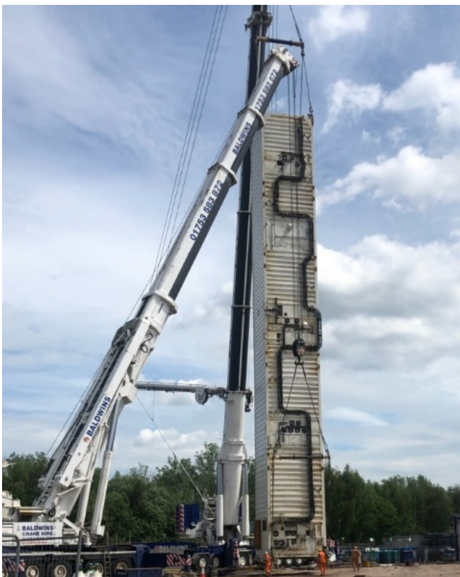
Lift of Rectification Tower in preparation for loading ready for transportation to Coleshill
